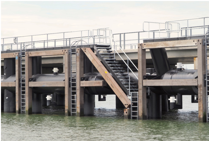
Berthing structure with traditional materials (courtesy: De Klerk Waterbouw)
